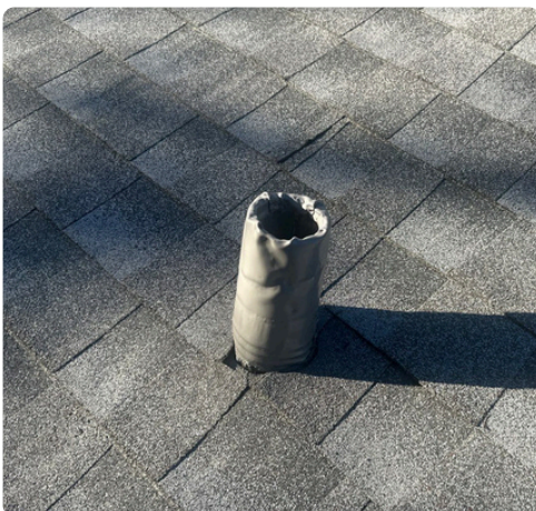
Pipe Flashing
